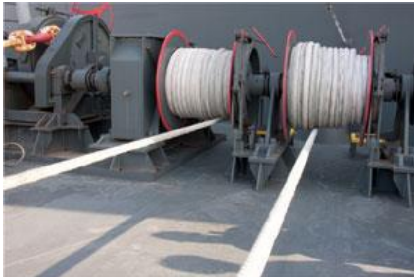
Fig. 9.2.B: Electric mooring winch and mooring lines (forward deck)
