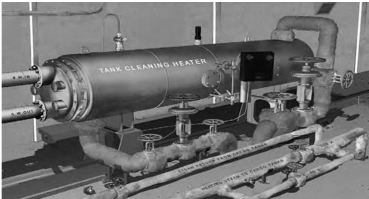
Fig. 7.3.4.B: Tank Cleaning heater
